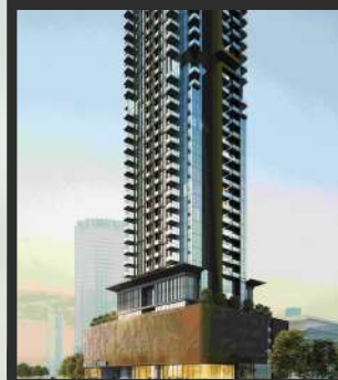
Seslia Tower JVT, Dubai
